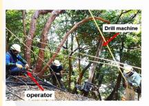
Slope protection technology to prevent landslide disasters that can achieve both forest protection and slope reinforcement. -Special drilling technology and surface protection technology enable slope protection work, such as soil nailing, without cutting down trees.
